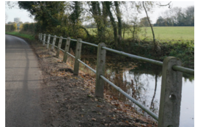
Concrete post and steel pole fence, which is not in keeping
