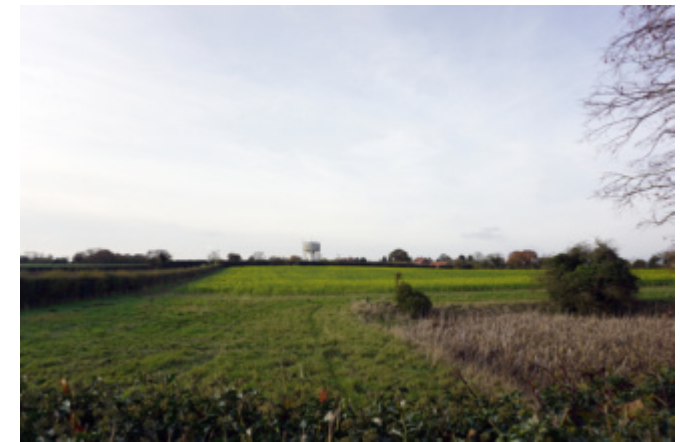
The water tower features in several views from within the Conservation Area
