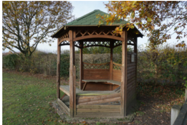
Damaged shelter at the playground
