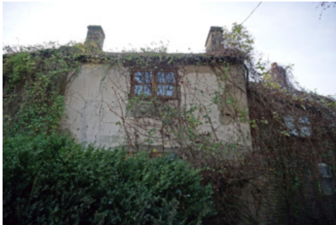
Cementitious render repairs
