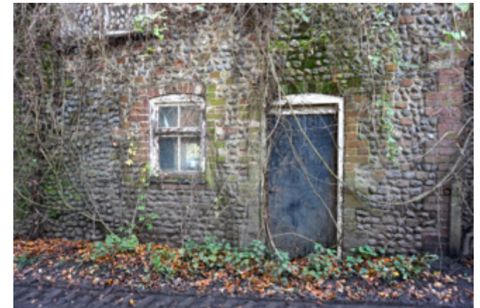
Timber work in poor condition
